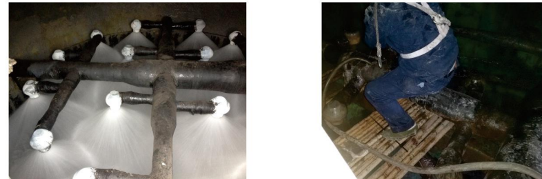
喷淋层疏通修复
